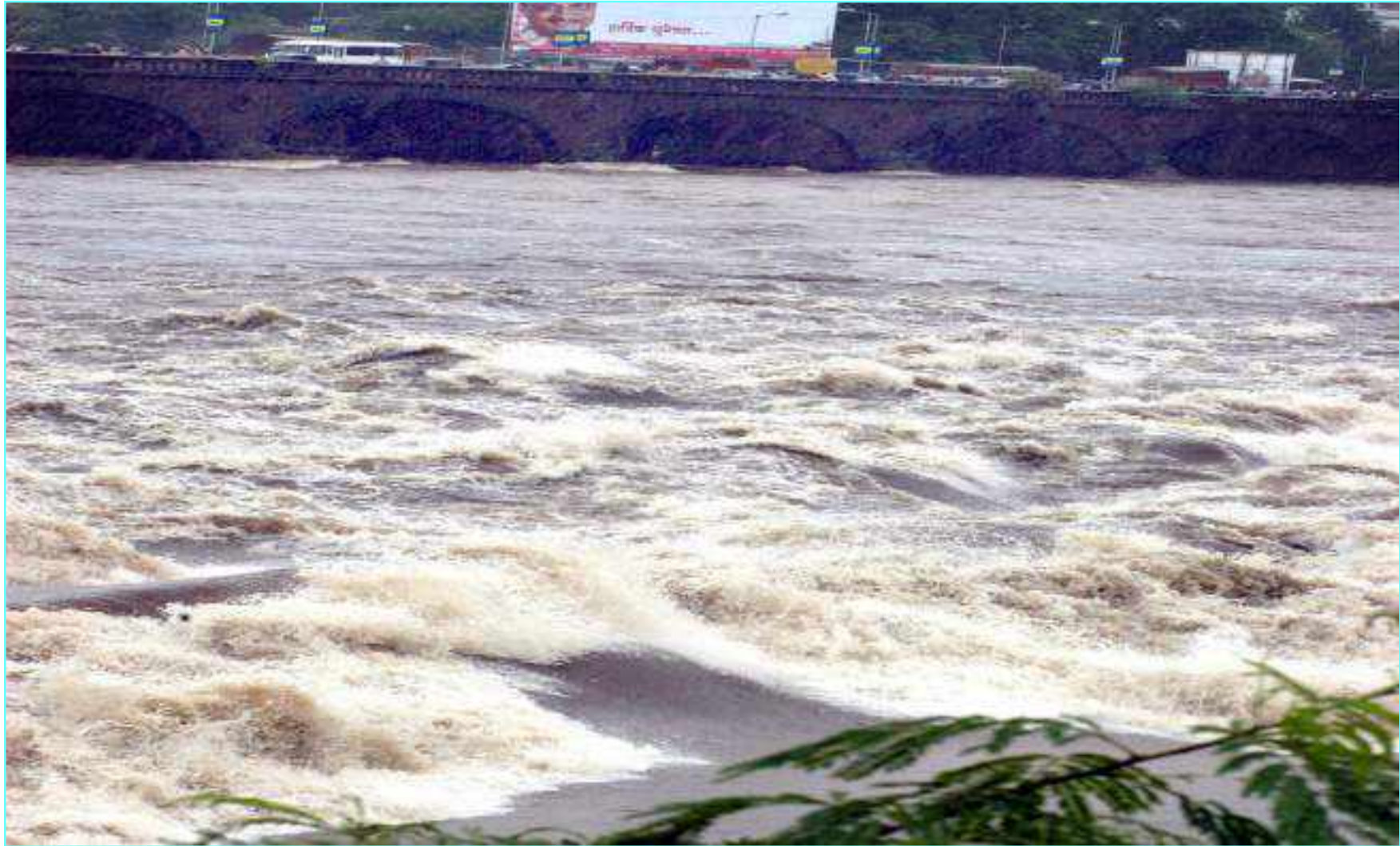
Flood situation at Shivaji Bridge, Pune
