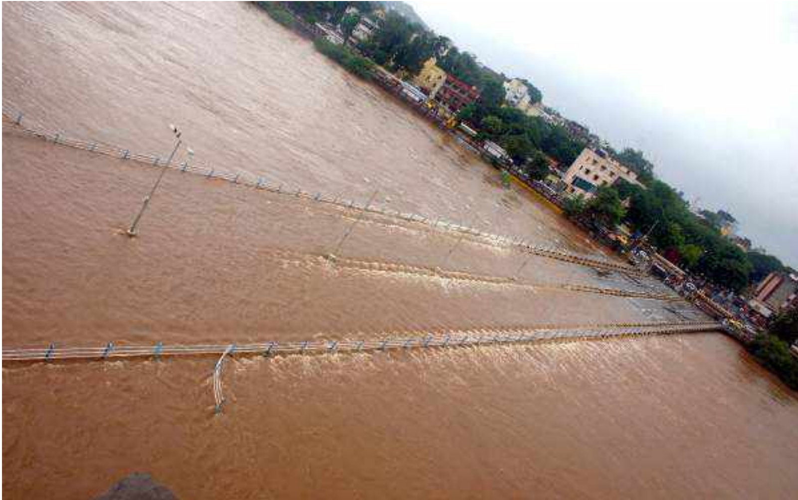
Flood situation at newly constructed Bridge near PMC
